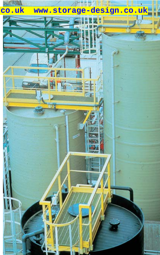
Liquid storage tanks with Allgrid flooring : 100% resistant to corrosion. (Allgrid on page 95).
