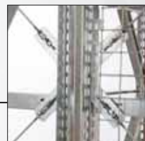
Back cross bracing with 4 point fixing
