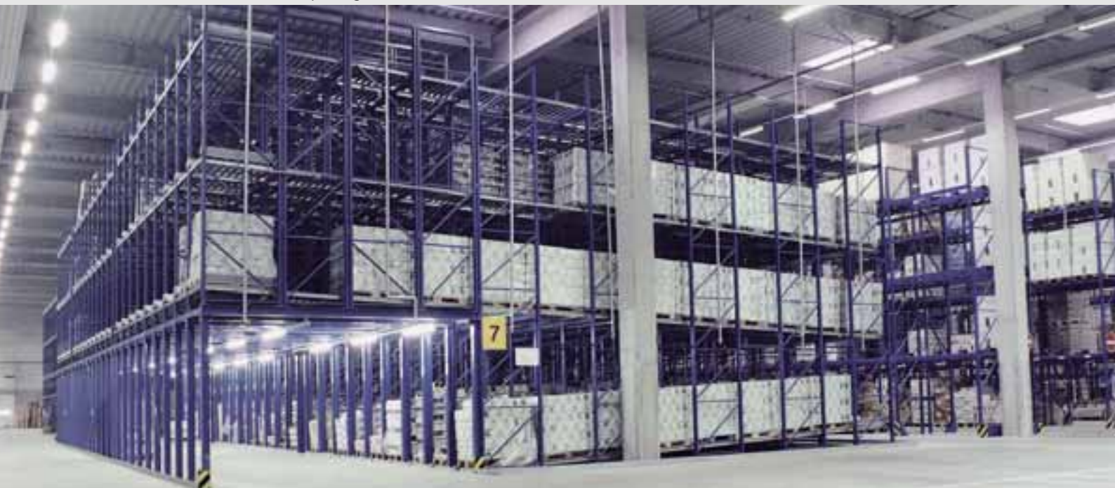
Goods distribution centre food with picking tunnel
