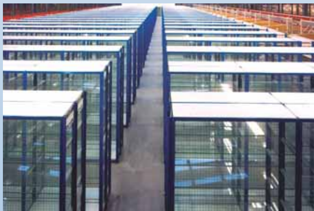
Single-tier QB2 in a Pharmaceutical Distribution Centre.
