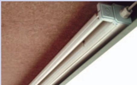
Under canopy light fitting complete with fluorescent tube.
