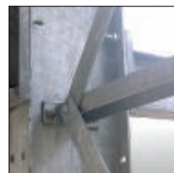
Detail of bracing connection on galvanised rack
