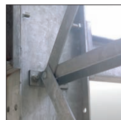
Detail of bracing connection on galvanised rack
