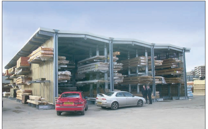
Continuous roof structure
